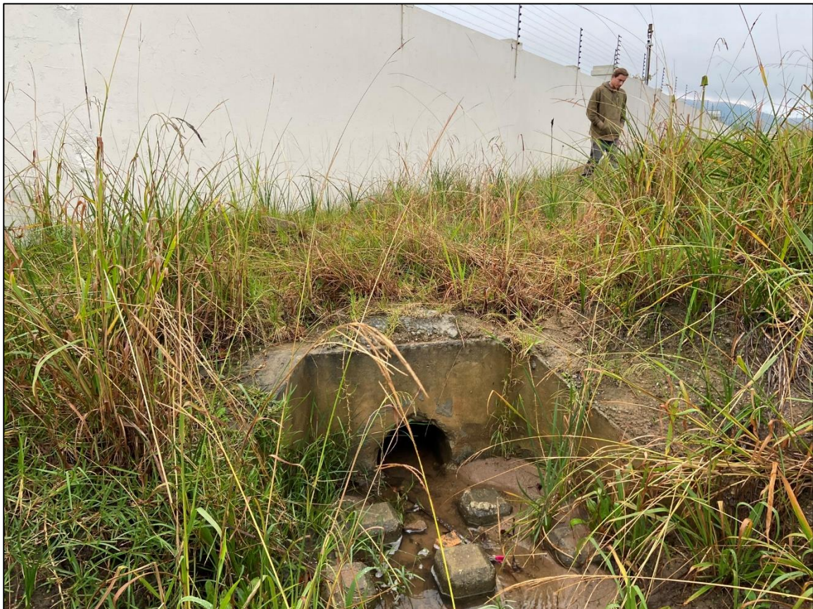
Figure 2: Image illustrating where the water enters the site through stormwater pipes along the northwestern border (June 2023).
