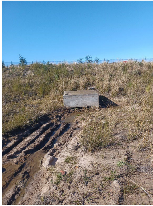
Figure 17 Stormwater drain in the south
