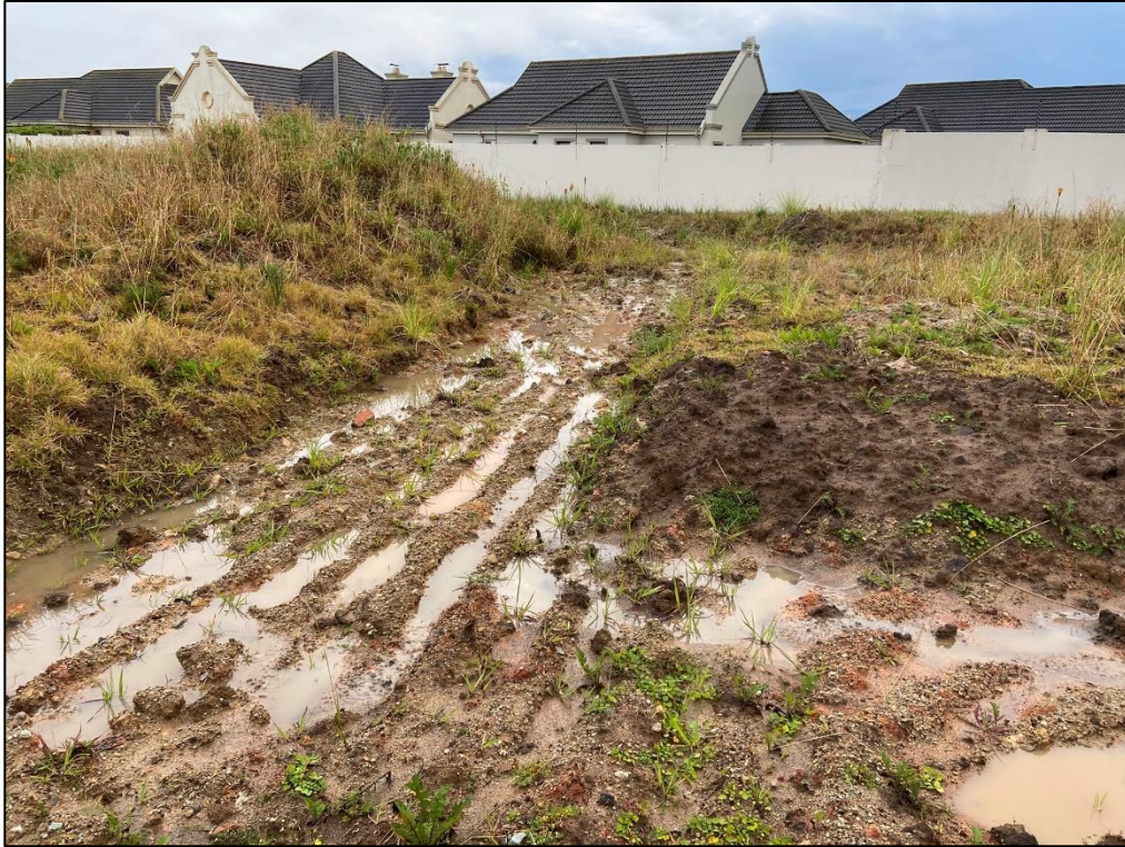
Figure 3: Image illustrating where furrows have been created to aid the drainage of stormwater on the site (June 2023).
