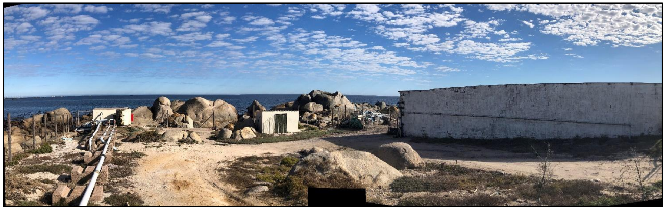
Inlet and outlet structures and crayfish holding building
