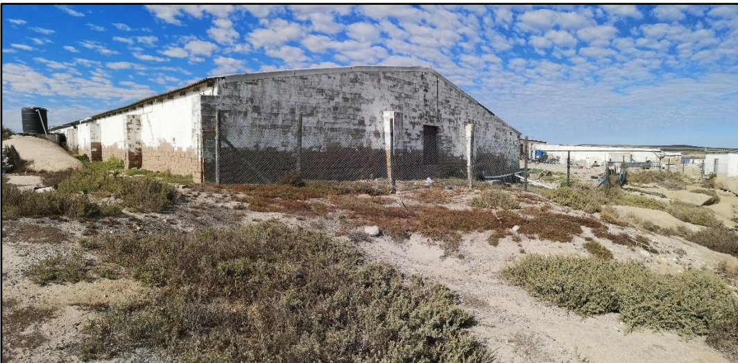
Buildings on Farm 1259 to be converted
