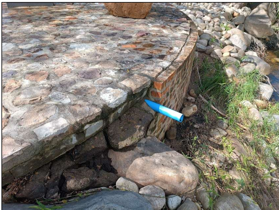
Figure 16: Photograph of the edge of a fire pit located within the watercourse. The blue pipe is an overflow for rainwater that accumulates in the pit.
