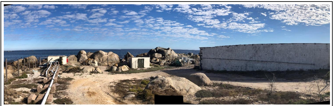
Figure 2: Site photograph showing the in and outlet structures and crayfish holding tank building
