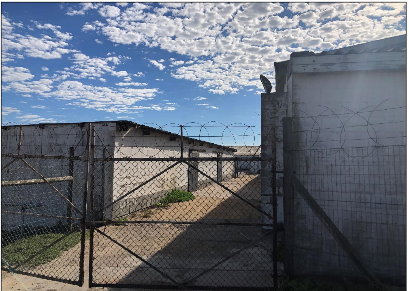
Figure 4: Existing buildings from the south
