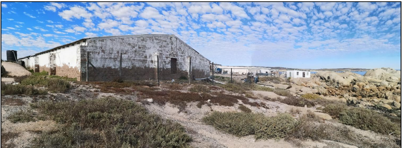
Figure 6: Existing buildings from the northwest
