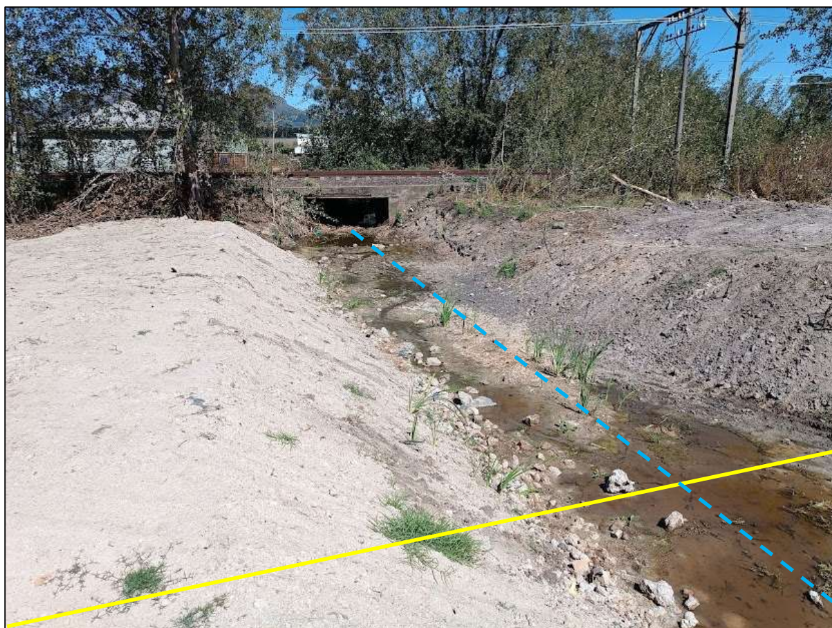
Figure 14: Photograph of the Sand River crossing site. The approximate alignment of the pipeline is indicated as a yellow line and the watercourse as a blue stippled line. Note the newly shaped banks and the extensive clearance of vegetation as well as the railway bridge located approximately 30m downstream of the proposed crossing point.
